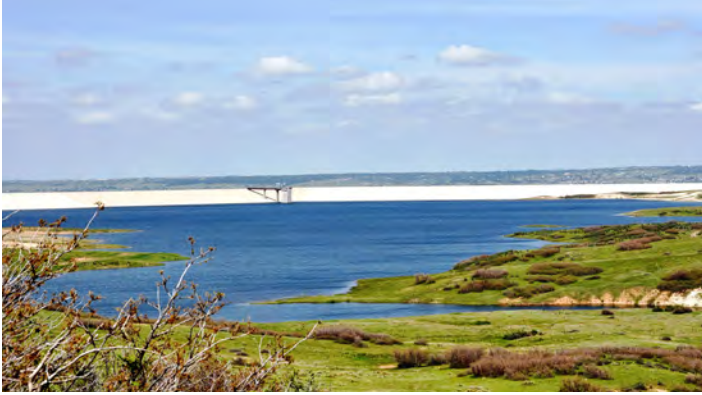
View of Rueter-Hess Reservoir ( www.pwsd.org )
